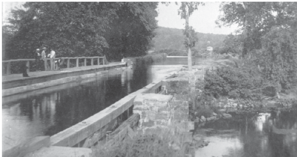
This historic view of Denville's Rockaway River Aqueduct shows the wooden trunk supported by three stone piers.
